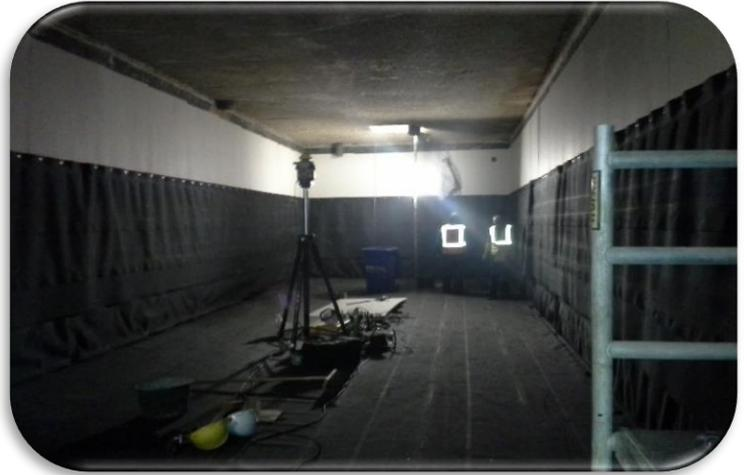
**VB-EPDM membranes** play a crucial role in making these basins watertight. The fact that the basins are often built indoors means their impermeability to water is of even greater importance.
