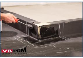
72. Gluing in membrane.
