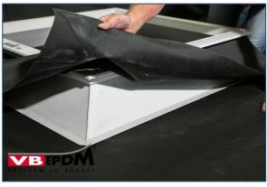
131. Positioning prefab sealing sleeve.
