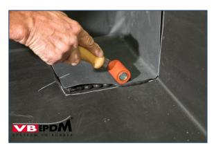
62. Roll the sealed part with silicone roller.
