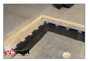
36. Reinforced EPDM strip as perimeter fastening.
