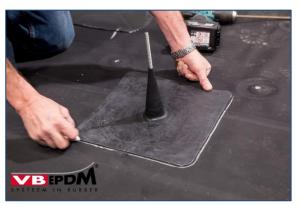
104. Positioning lightning conductor sealing sleeve.
