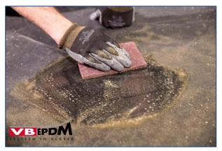
159. Cleaning place of the repairs.
