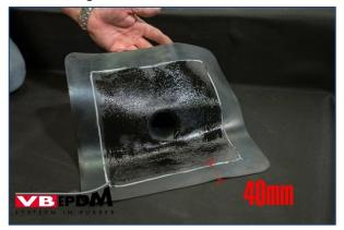
144. Gluing in flashing VB drain.
