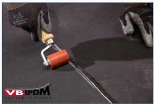
166. Rolling repair piece with silicone roller.
