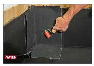
60. Rolling sealing sleeve with silicone roller.
