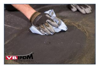
160. Rubbing place of the repairs dry.
