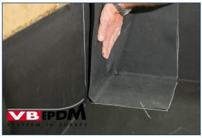
59. Rubbing sealing sleeve with flat hand.
