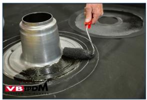
90. Gluing in substrate.
