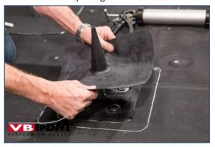
107. Placing lightning conductor sealing sleeve.
