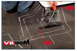
123. Gluing in membrane.
