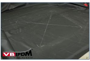
112. Cutting into membrane (**Note protection against falling!**).
