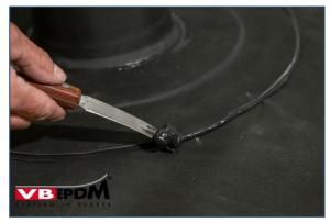
101. Remove excess sealant with blade.
