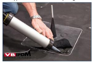
108. Sealing the sealing sleeve with VB-9510.
