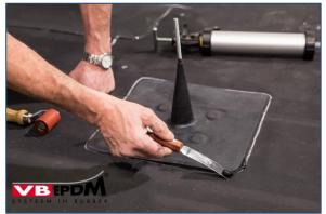
110. Removal of excessive sealant.
