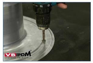
84. Mechanically fixing lead-through.
