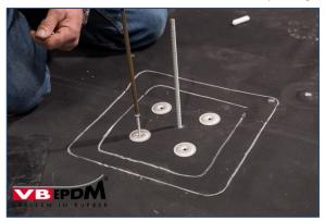
105. Mechanically fixing membrane.
