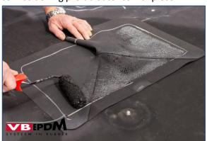
71. Gluing in prefab outer corner piece.
