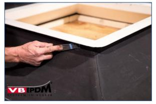
136. Folding shut sealing sleeve edge.
