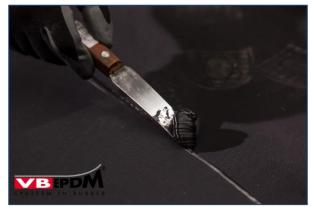
167. Removal of excessive sealant.
