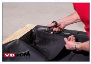
39. Cutting in inner corner with scissors.
