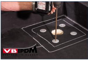
141. Mechanically fixing membrane.
