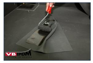
57. Gluing in sealing sleeve.
