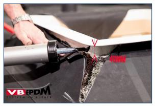
121. Sealing top side of membrane with VB-9510.
