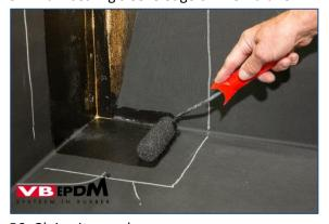
56. Gluing in membrane.
