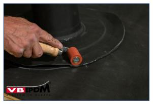
100. Rolling seal seam with silicone roller.
