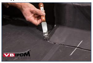
79. Remove excess sealant with blade.
