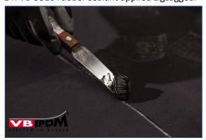
26. Remove emerging rubber sealant.
