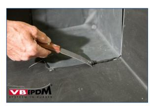
63. Remove emerging excess rubber adhesive.
