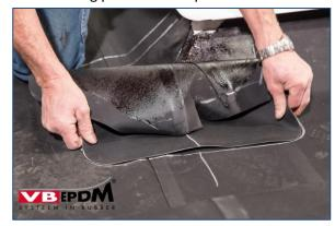
124. Placing prefab corner piece.
