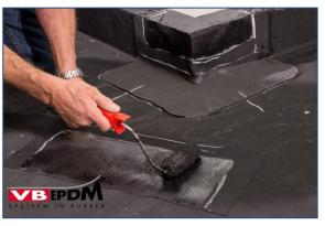
81. Gluing in corner sealing sleeve and substrate.
