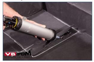
145. Sealing flashing with VB-9510.
