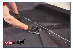
22. Folding VB-EPDM seam joint shut.
