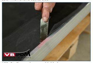
155. Sealing seal seam with blade.
