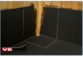
55. Sealing sleeve position marked on membrane.
