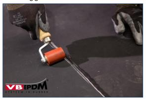
25. Rolling adhesive/sealant seam with silicone roller.
