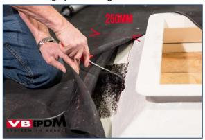
117. Gluing in dome upstand.
