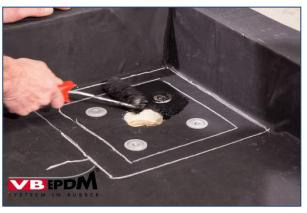
143. Gluing in membrane.
