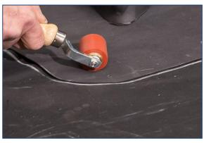
23. Rolling glued seam with silicone roller.
