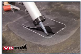
165. Sealing repair piece with VB-9510.
