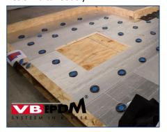
5. Thermofix® elements fastened.
