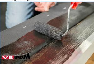
149. Gluing in roof trim + membrane.
