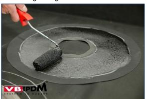
89. Gluing in sealing sleeve.
