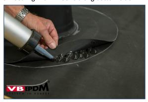
99. Sealing with VB-9510 in the roof plane.
