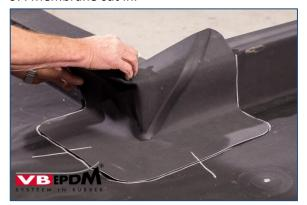
69. Positioning prefab outer corner piece.
