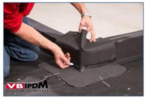
80. Marking upper part corner sealing sleeve.
