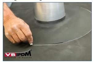
87. Marking sealing sleeve on membrane.
