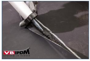
24. VB-9510 rubber sealant applied zigzagged.
