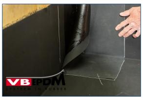
58. Fitting sealing sleeve.
