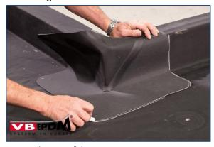
68. Marking prefab outer corner piece.
