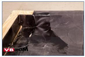
37. Glued-in roof elevation at inner corner.
