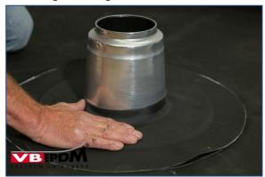
91. Placing sealing sleeve.
